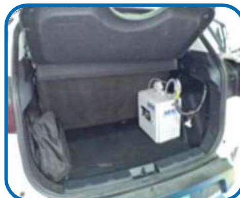
Controller Mounted in Vehicle Boot
