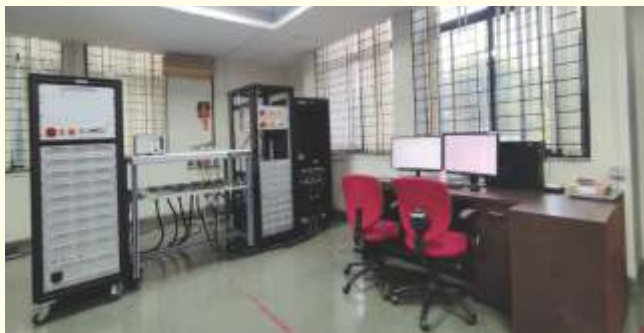
300 V EV HIL System with Start-up BMS at Pune
