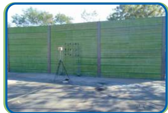
Noise Barrier in-situ Acoustic Performance as per EN 1793 – Part 4, 5, 6
